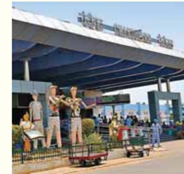
Chandigarh Railway Station
